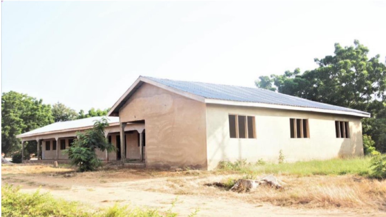
CONSTRUCTION OF 1 NO. 3 UNIT CLASSROOM BLOCK AT GYAKITI-DACF
