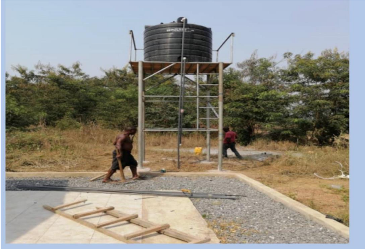
CONSTRUCTION OF 1 NO. BOREHOLE AT AKRADE- DACF/RFG
