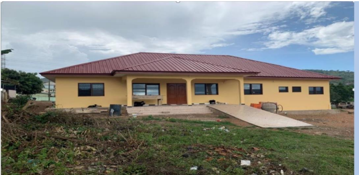
CONSTRUCTION OF CHPS COMPOUND AT AKRADE – DACF
